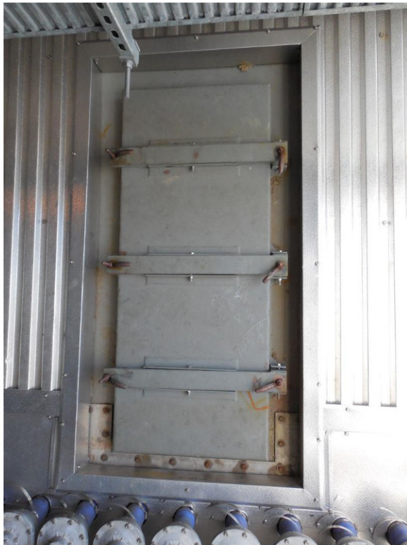
Walk in Plenum with insulated entry door
